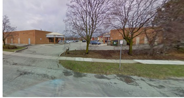
Figure 2-3: Eastern view of 501 Krug
