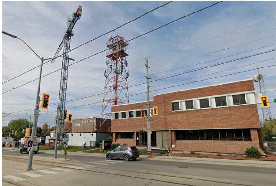
Figure 2.1 - Existing office building long King Street West
