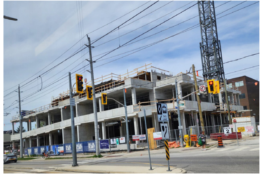
Figure 2.11 - Multi-residential development under construction west across Pine Street
