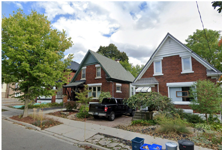
Figure 2.10 - Low-rise residential neighbourhood between Park Street and York Street
