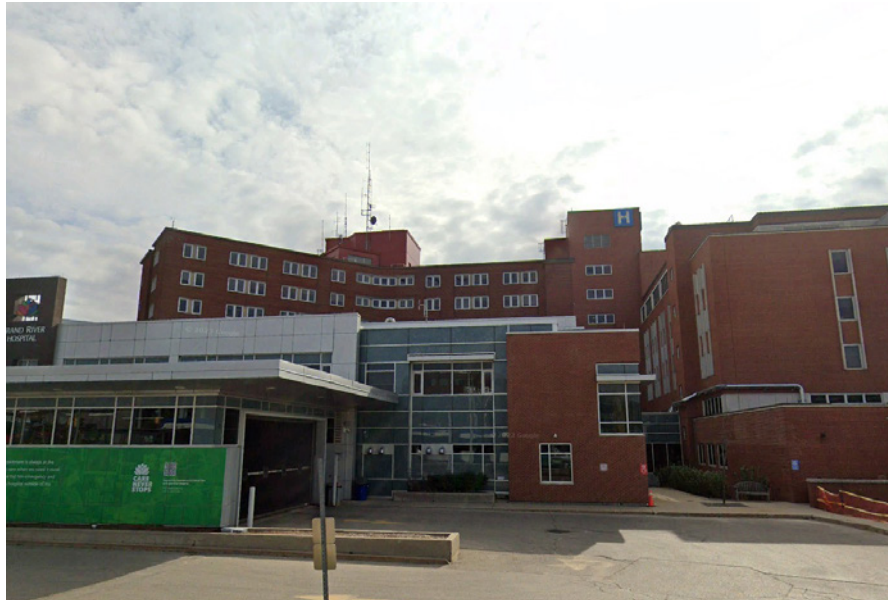
Figure 2.9 - Grand River Hospital south across the Site
