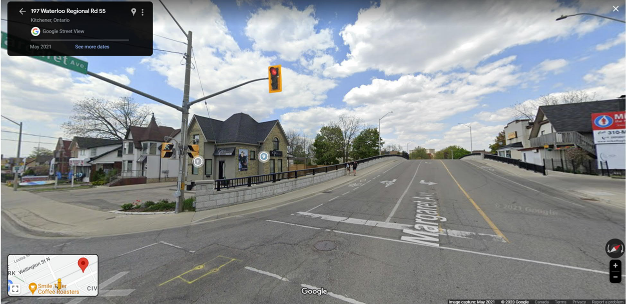
Figure 4: Looking Towards Guelph Subdivision at Corner of Victoria Street North and Margaret Avenue, West of the Proposed Development
