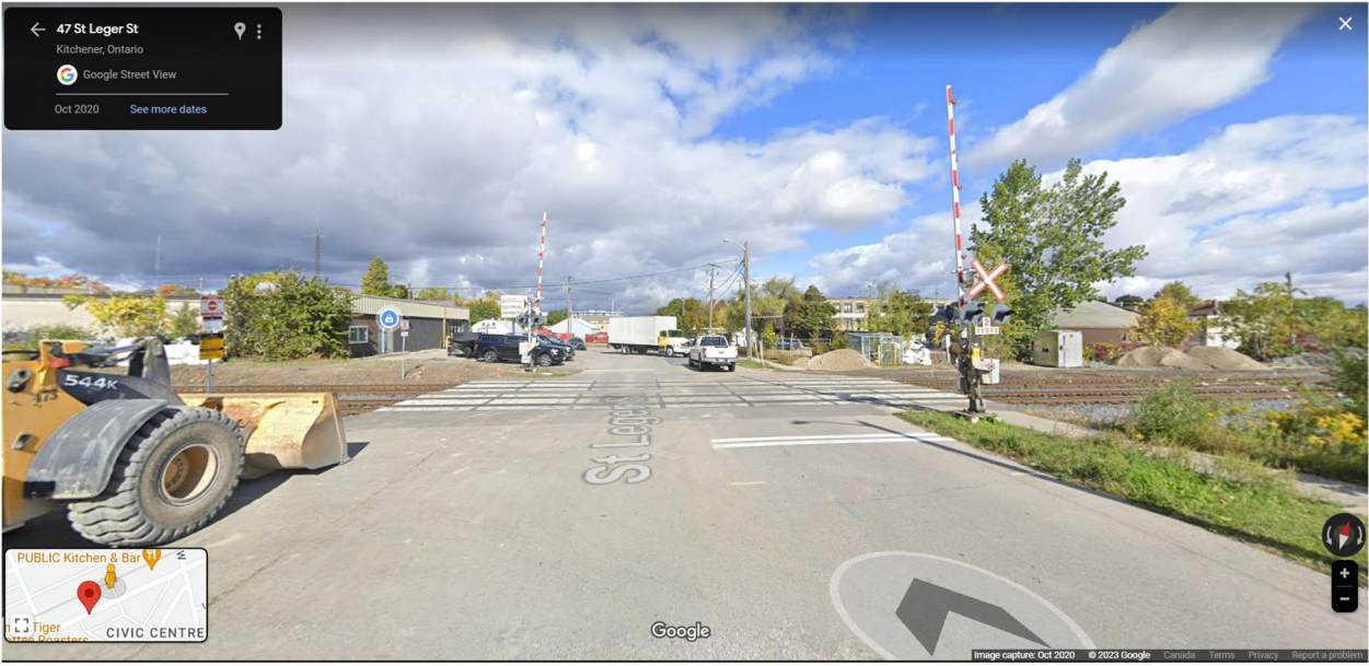
Figure 5: Looking Towards Guelph Subdivision from St Leger Street, East of the Proposed Development
