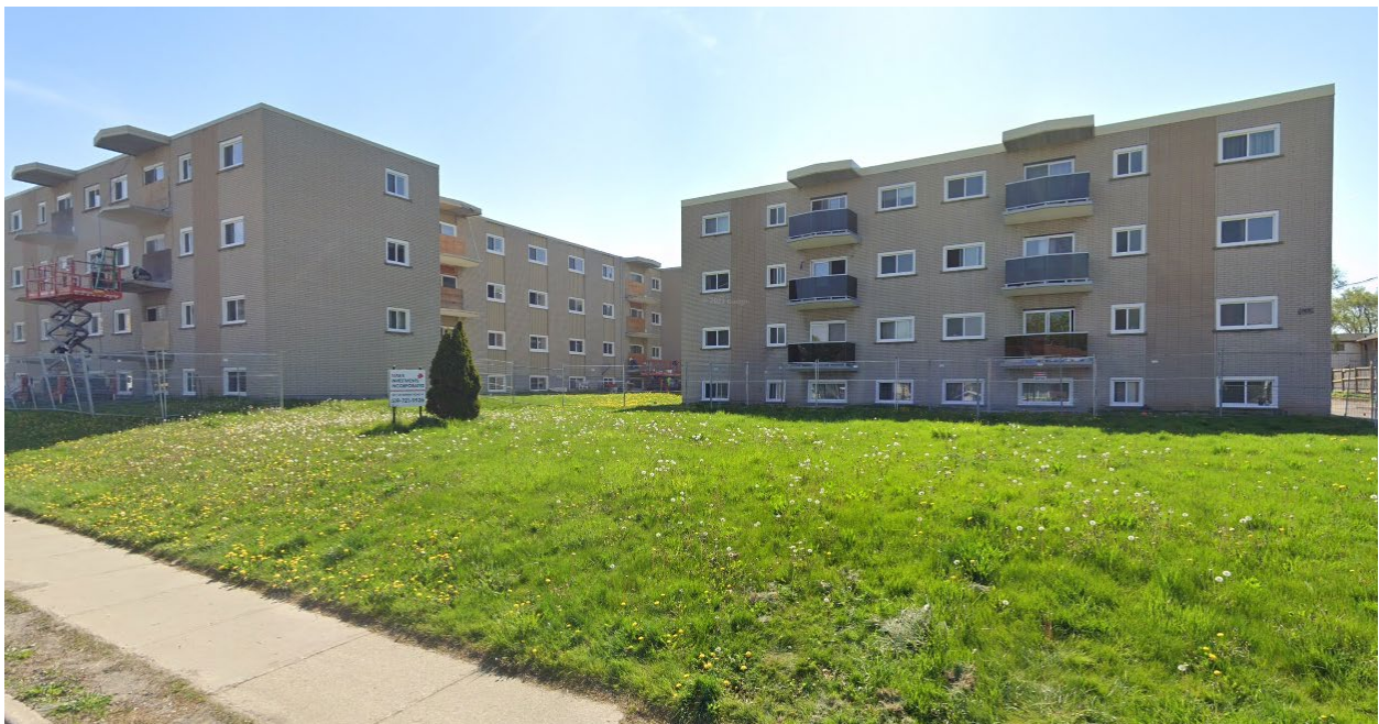
Figure 14: Apartment Complex at 149 Fairway Road (Source: Google Streetview)
