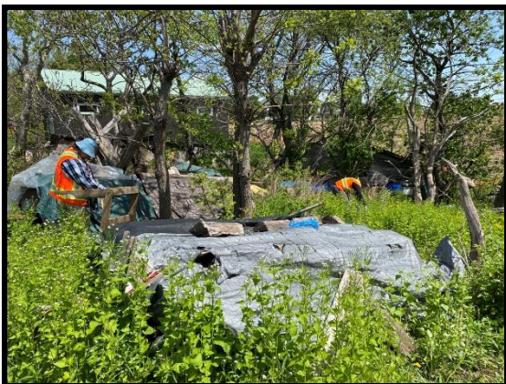
Image 9: Test Pit Survey (May 24, 2022; Facing Northeast)
