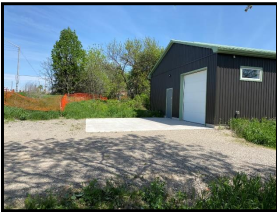
Image 3: Disturbed Lands (May 24, 2022; Facing Northeast)
