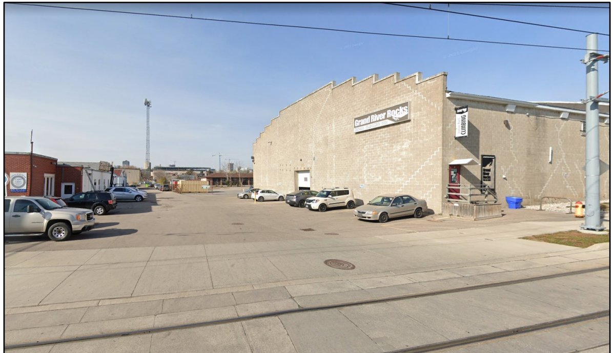
Figure 5: Streetview of the Existing Access, facing West from Borden Avenue South (Source: Google Maps)
