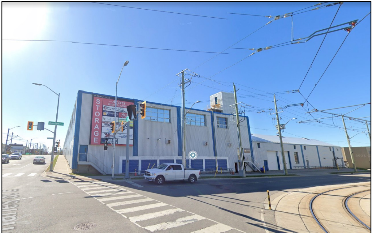
Figure 8: Commercial Development, 50 Ottawa Street South facing Southeast from Charles Street East (Source: Google Maps)
