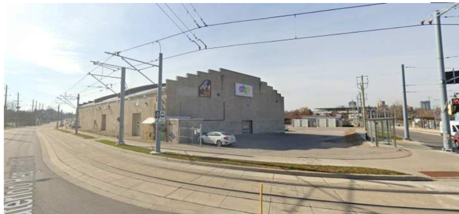
SITE CONTEXT / VIEW FROM BORDEN AVE S
