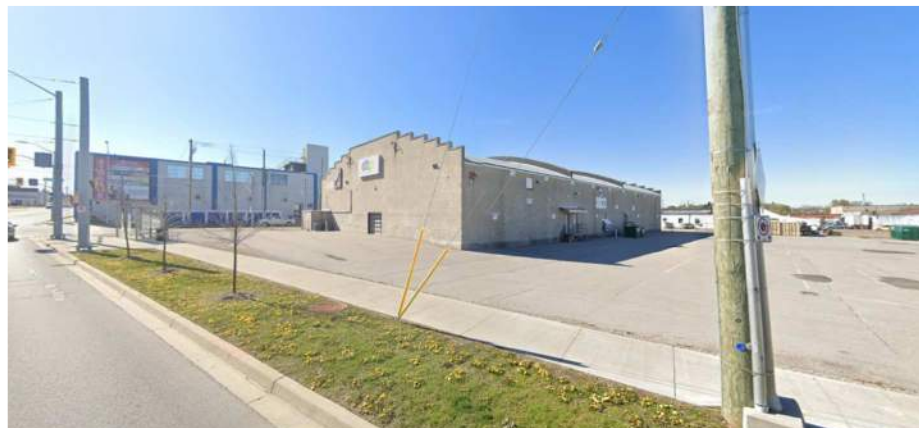
SITE CONTEXT / VIEW FROM CHARLES ST E
