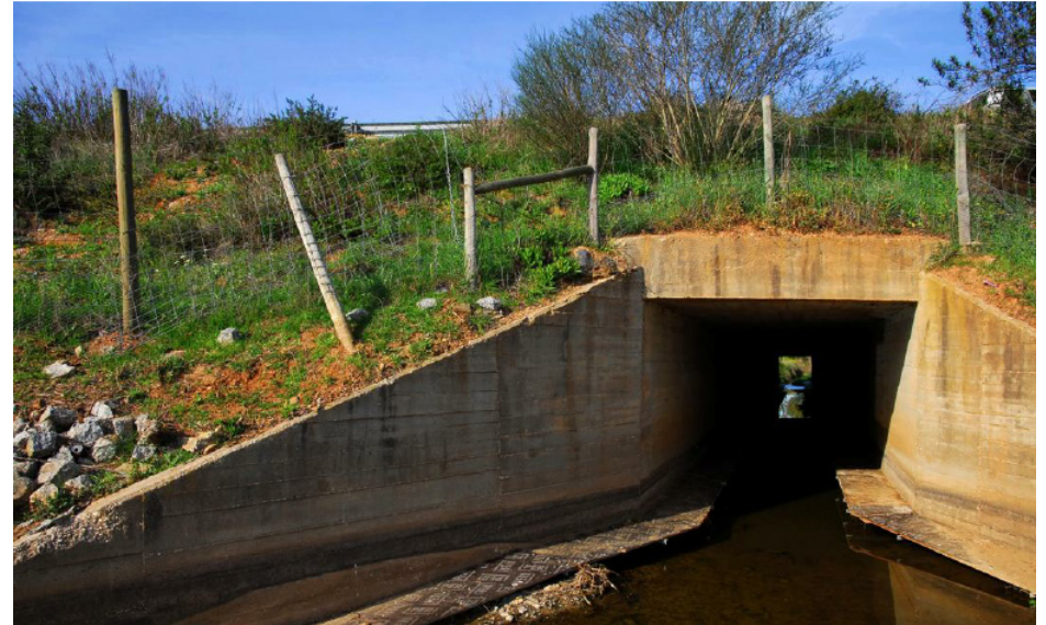
Example of a box culvert for passage of small animals
