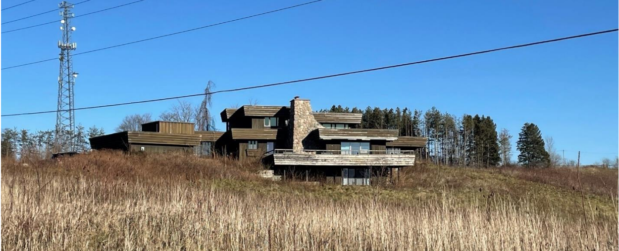
Figure 3: View of the Shantz House from Trussler Road (looking east)
