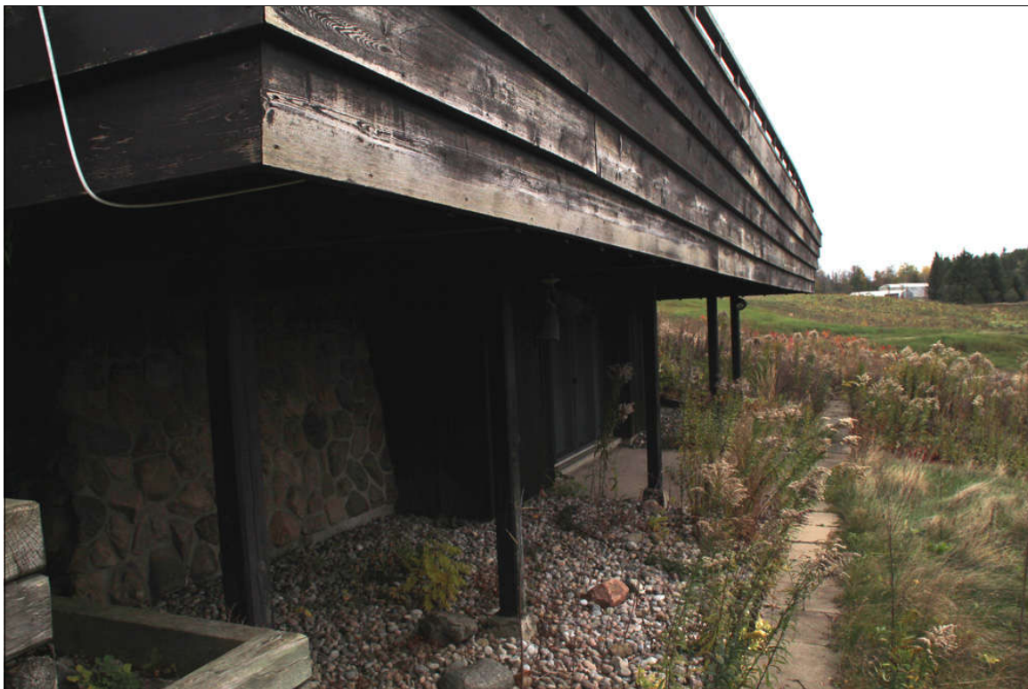
Figure 37 underside of deck at south end
