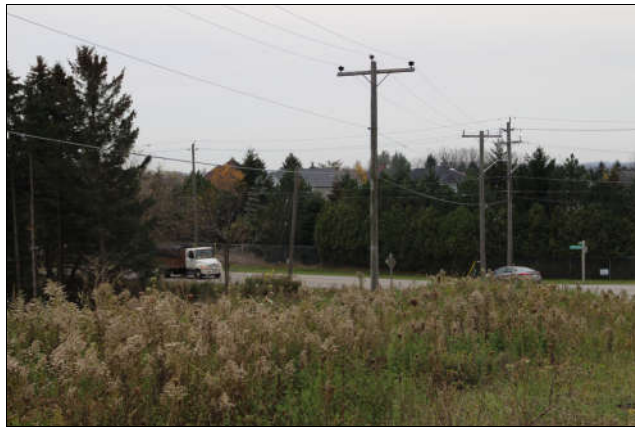
Figure 21 view southwest to Trussler Road
