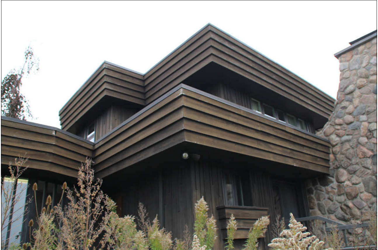
Figure 38 cedar fascia board, board & batten siding, fieldstone chimney tower - west elevation
