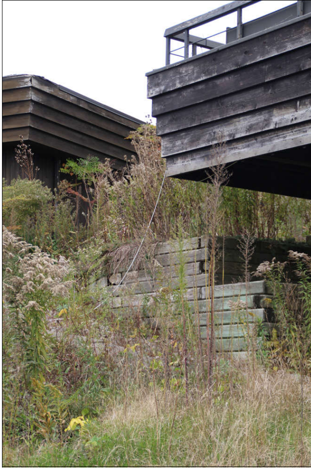
Figure 35 timber retaining wall
