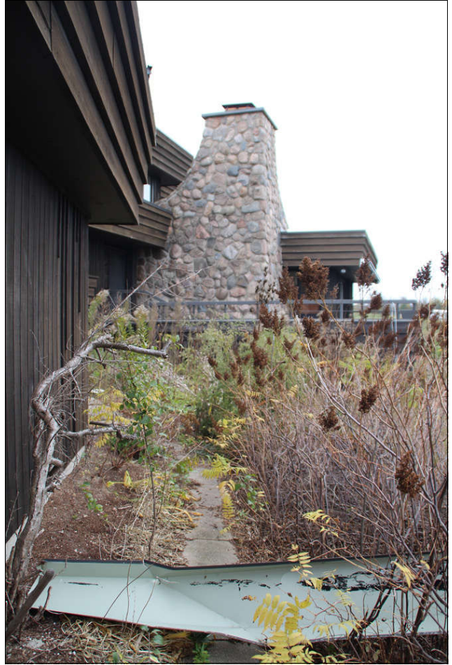
Figure 36 west side landscape, precast concrete walk
