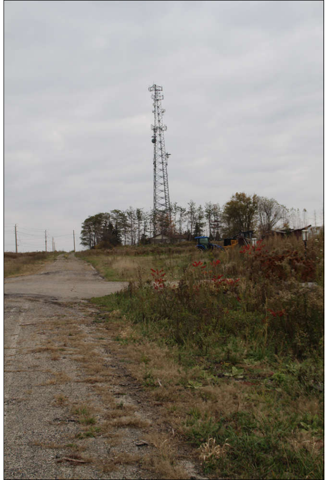
Figure 26 communications tower east of house old Mannheim Road roadbed remnant
