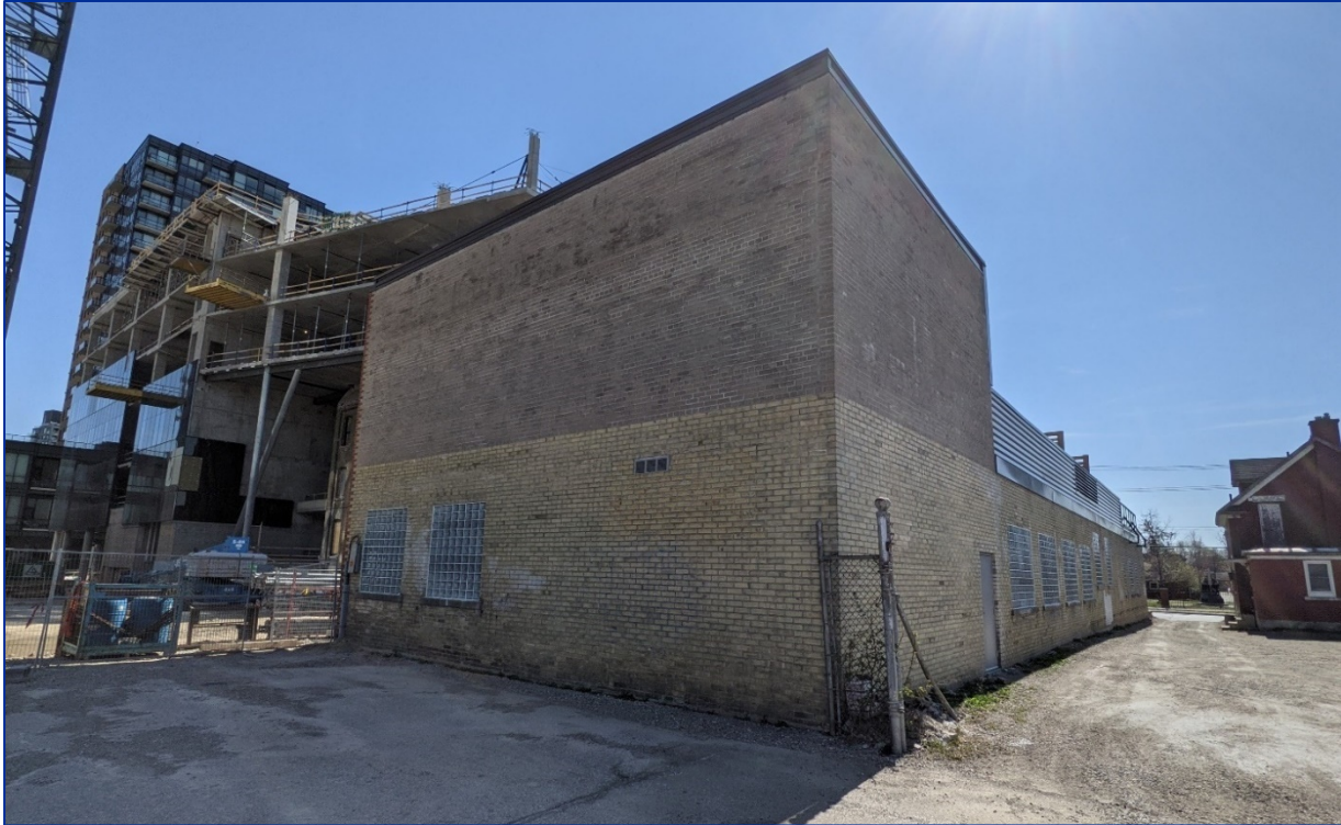
Figure 21: View southeast of northwest and southwest elevations
