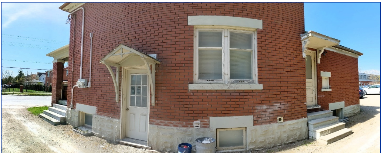
Figure 25: Panoramic view of northeast elevation
