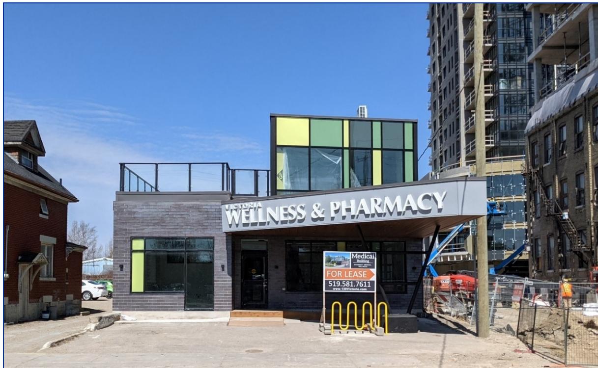
Figure 14: View northwest of southeast façade
