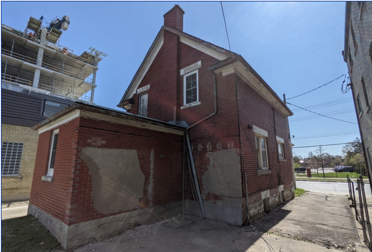
Figure 27: View northwest of northwest elevation and southwest elevations
