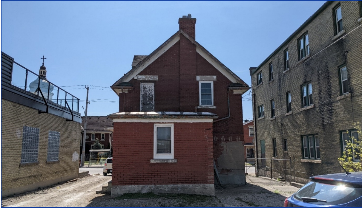
Figure 26: View southwest of northwest elevation
