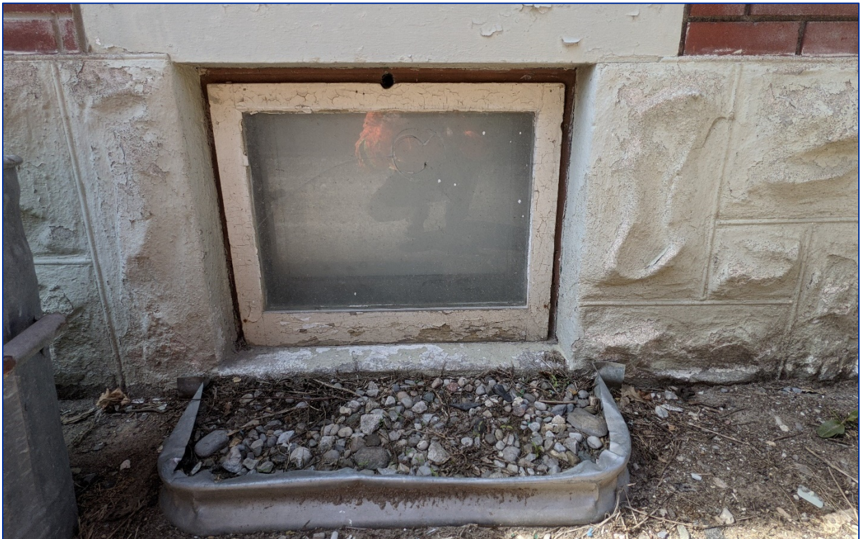
Figure 29: View of northeast basement window
