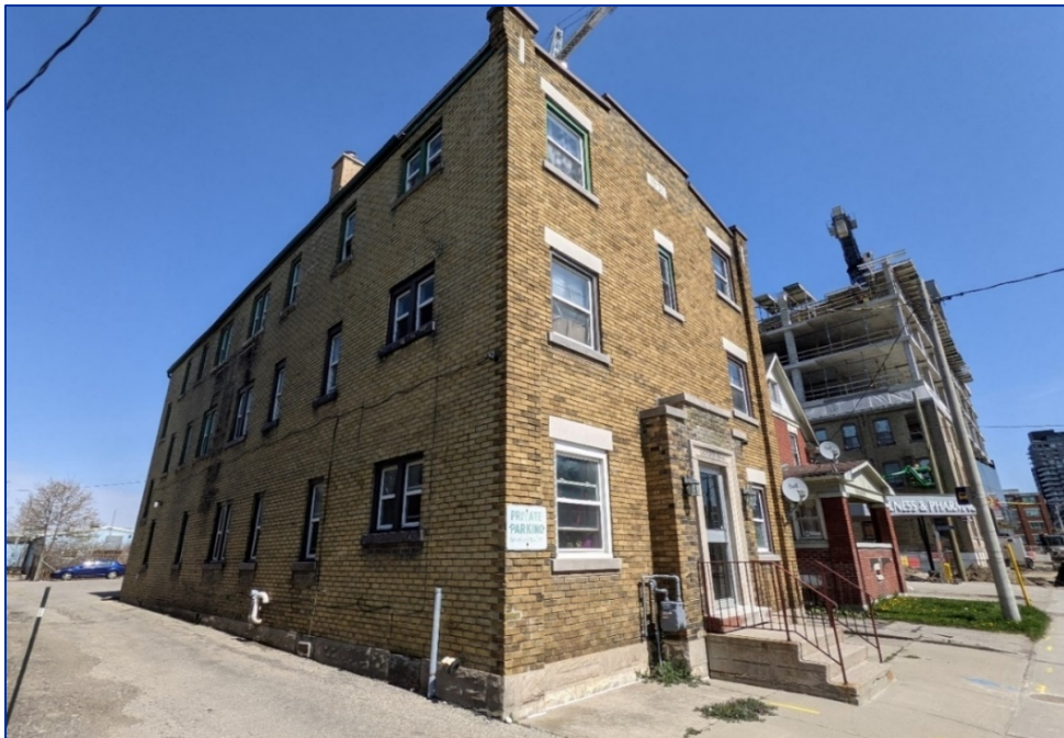
Figure 33: View northwest of southwest corner
