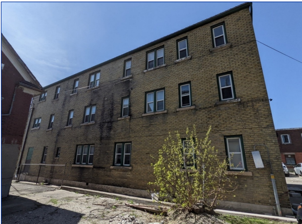
Figure 35: View southwest of northeast elevation
