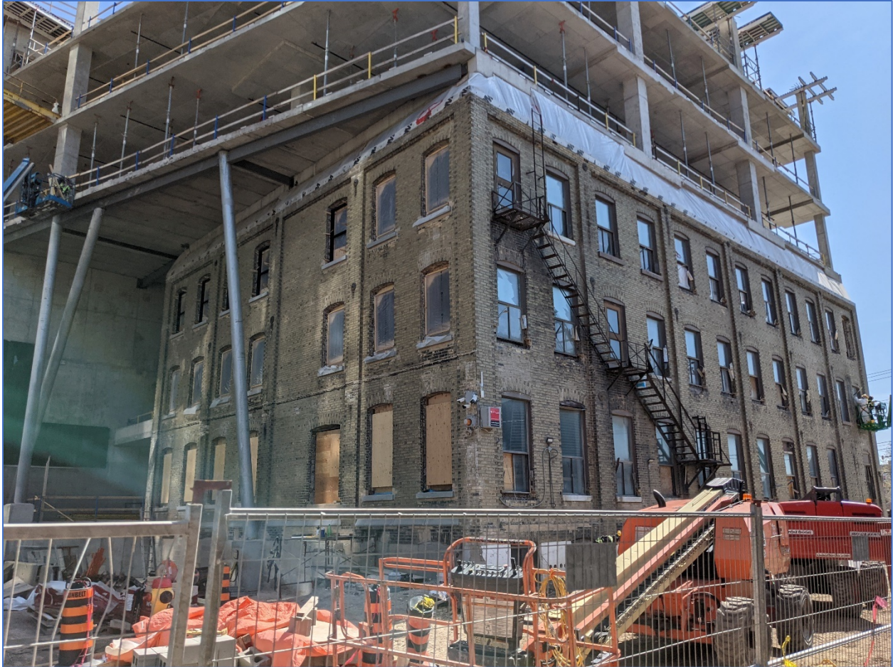
Figure 50: View northeast of the northwest and southwest elevations of 120 Victoria Street
