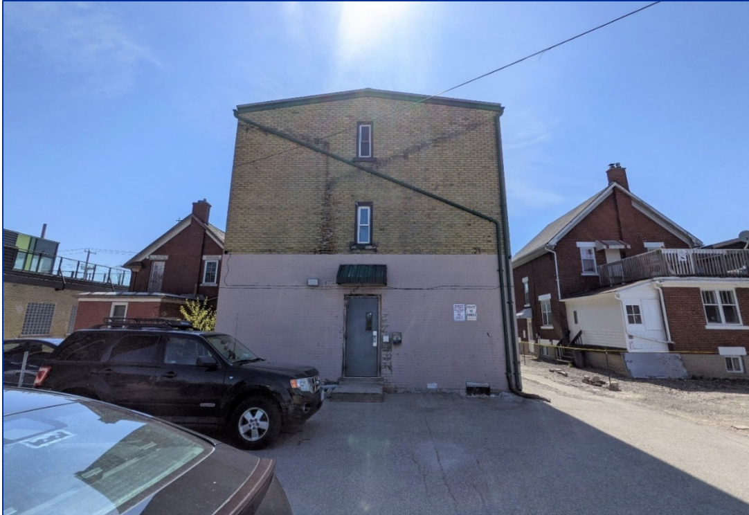
Figure 36: View southwest of northwest elevation
