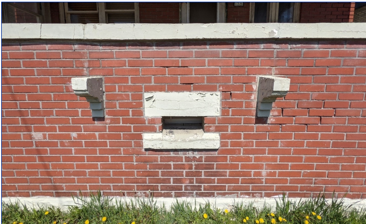
Figure 31: View northeast of porch brackets and opening
