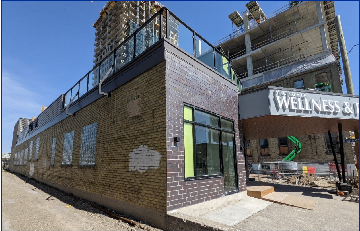
Figure 23: View northeast of southwest and southeast elevation
