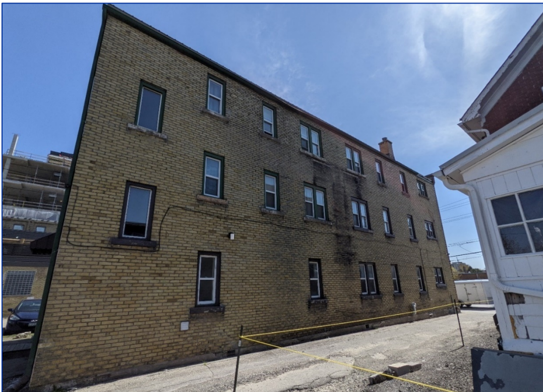
Figure 37: View southeast of southwest elevation
