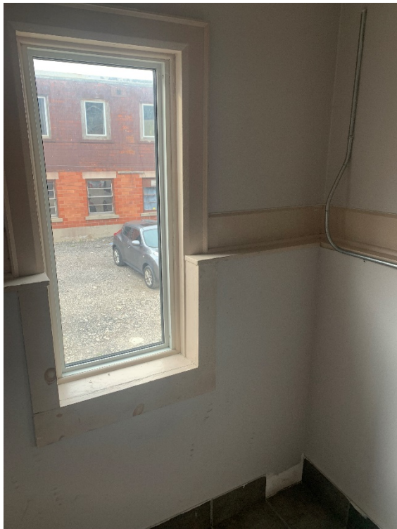
Figure 43: Window in rear stair well
