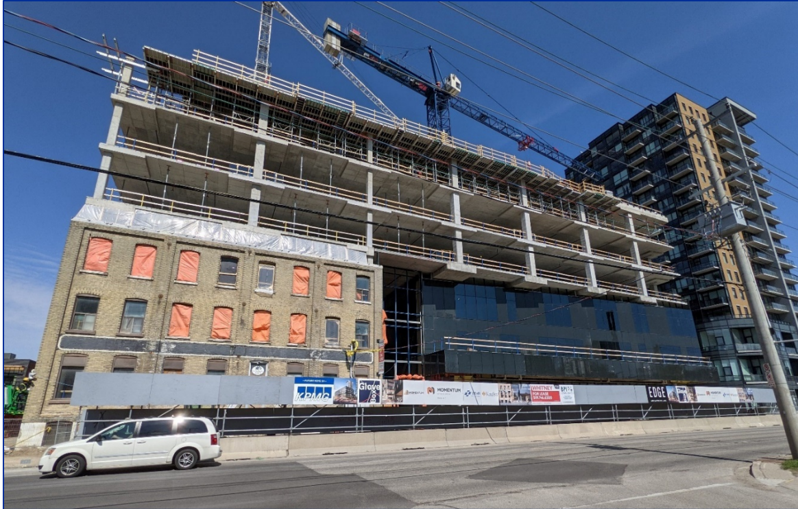
Figure 46: View of adjacent development
