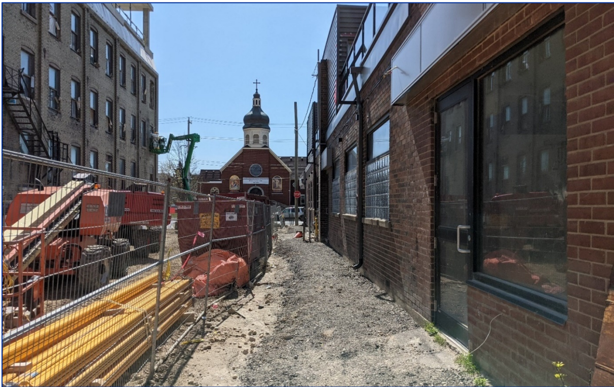
Figure 18: View southeast of northeast elevation
