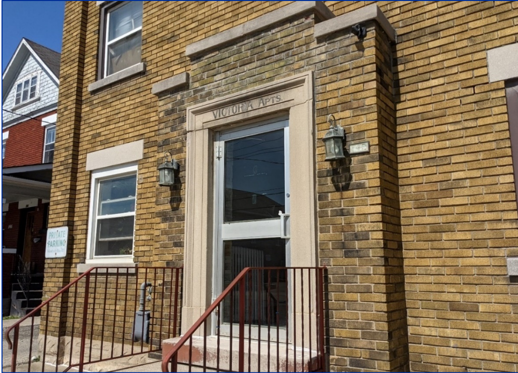
Figure 34: View of main entrance
