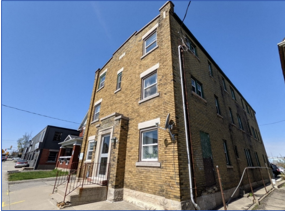
Figure 32: View southwest of southeast façade
