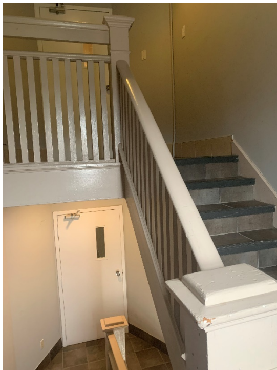
Figure 39: Interior, front stairs
