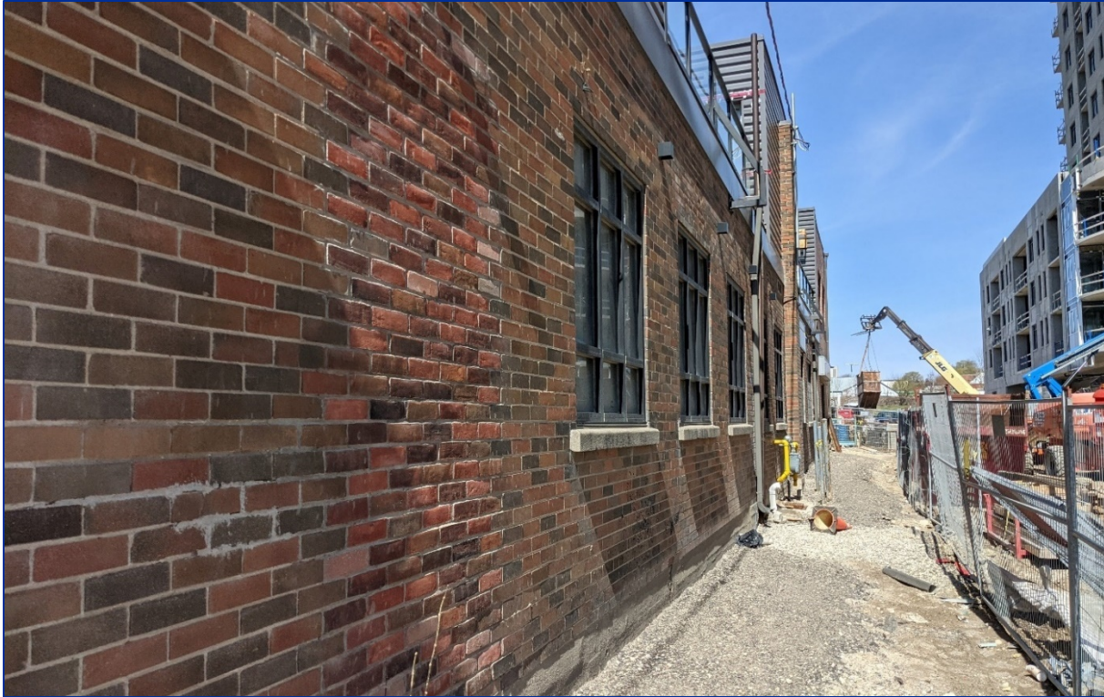
Figure 17: View northwest of northeast elevation
