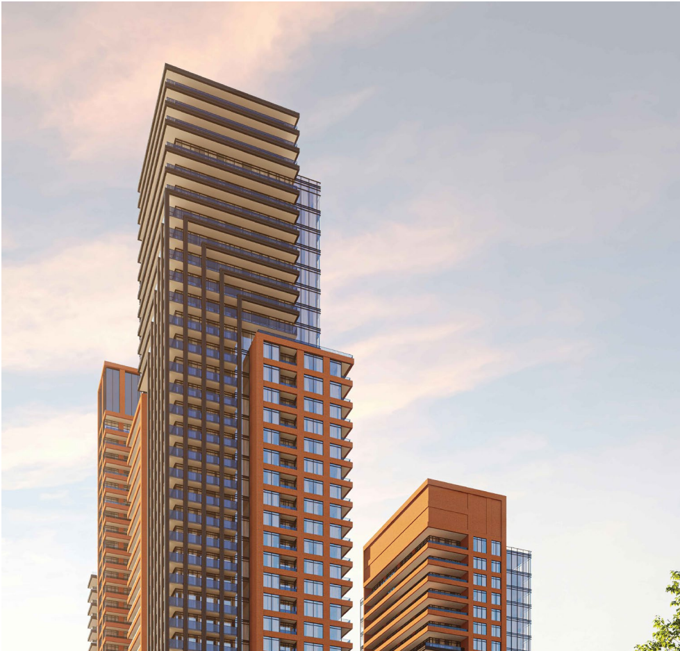
IMAGES: Rendering of proposed development distinct tower top treatments of materials, colour and balconies (Source: IBI Group, adapted).
