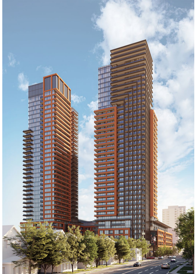
IMAGE: Rendering of proposed development looking east along Victoria Street South (Source: IBI Group).
