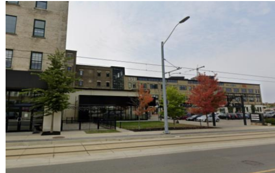
Tannery Building, iON rail (South)
