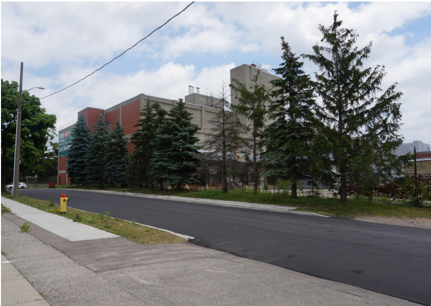
Palmer Avenue Streetscape
