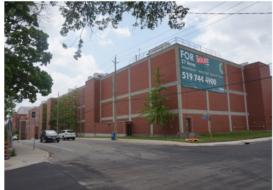
Former Plant Building on Courtland Avenue East
