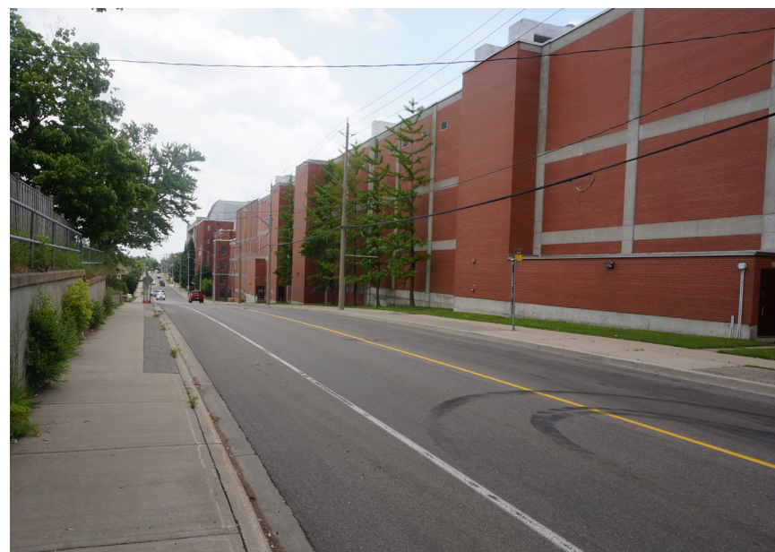
Courtland Avenue East Streetscape (pre-demolition)
